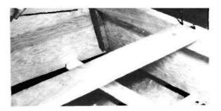
Chine goes into notch cut for it in transom. Note the two screws joining the inner keel to transom.
