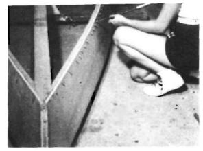
Ratchet screwdriver makes short work of setting the screws; no linen strips are used on the glued side joint since chine face is milled at factory.
