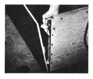
After drilling the sides for screws, glue them to the transom batten. Into the glue bed, lay linen strip which compresses, distributing the Weldwood marine glue entirely over the surfaces.
