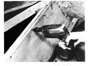
With %-inch No. 7 Screwmate, predrill all holes for all panels two inches apart, as shown in photo.
