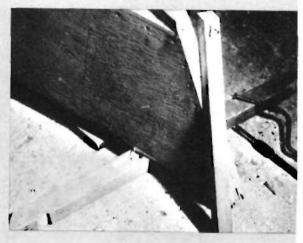
The final touch for the nose is the outer stem It will be planed to a taper after screwed into place.
