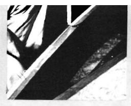
Linen strips are laid into Weldwood glue before securing bottom. Again compress glue onto surface.
