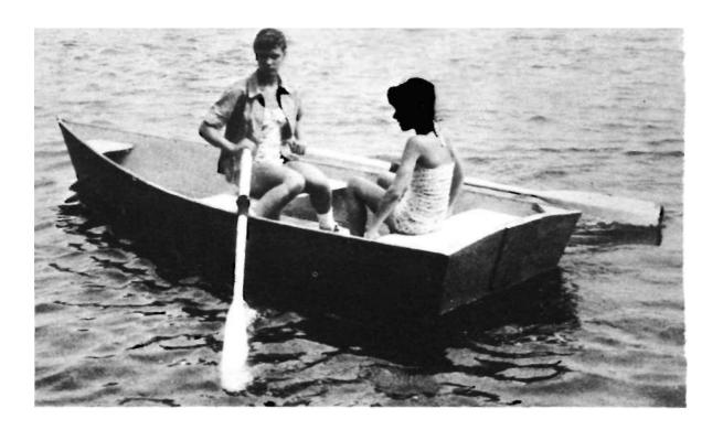
THIS 11-foot hull will cost you only \$35 to build and comes out of a single sheet of %-inch plywood. We used Weldwood Royal Marine Plywood for the job. It can be put together by almost any workshopper with a minimum amount of tools and time.
