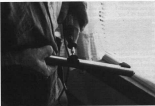
If no milling machine is available, slots and openings can be cut with a hand grinder using cut-off wheels.
