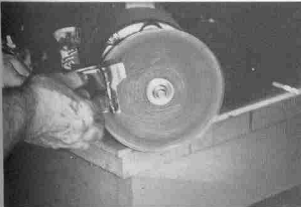
Welds are ground flush with disk sander.
